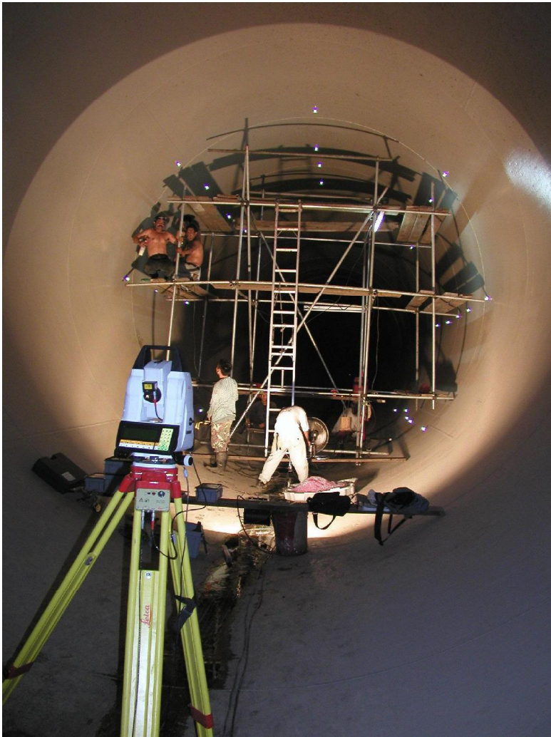
Picture 3: Internal surveying, typical set up for the total station theodolite method
