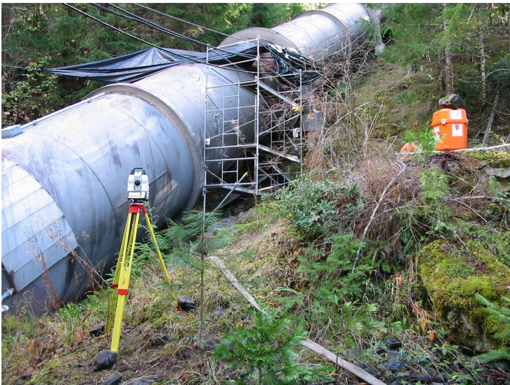
Picture 1: Typical set up for the mechanical theodolite method (courtesy of Accusonic Technologies, Jim Walsh)
