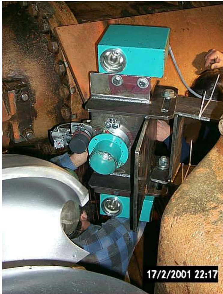
Figure 1 - Mounted instrumentation within the turbine housing in the shelter of the injector five and its deflector
