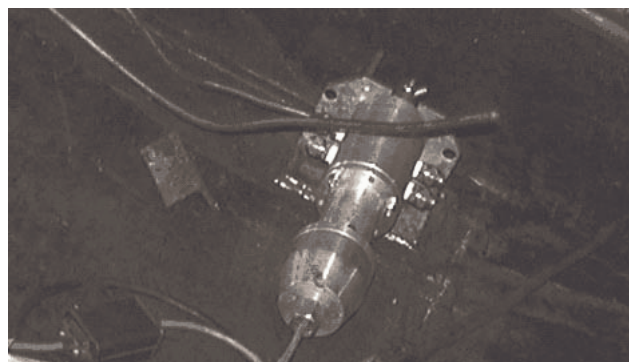
Fig. 9. View of the manifold installed in measuring section 1-1, with the absolute pressure transducer mounted inside.
