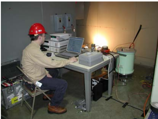
Figure 1 - PT Calibration Testing at Grand Coulee Powerplant (Computer and DMM shown on table, standard PT located behind table.)
