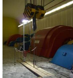
Fig. 10: Crane lifting the pipe frame within the bulkhead gate
