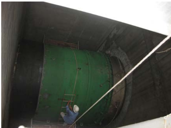
Fig. III. Installation of UTTF
