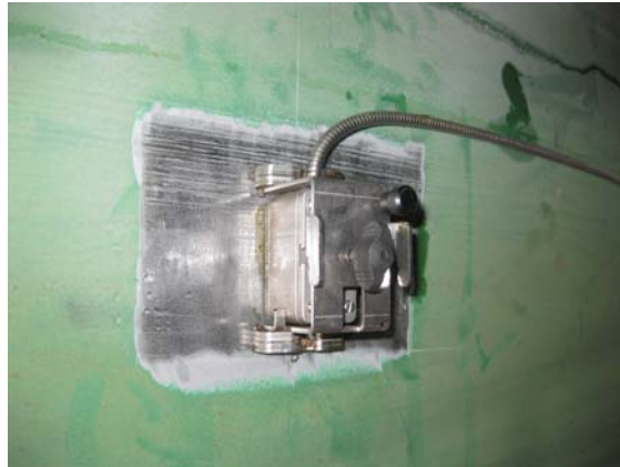
Fig. IV: Surface Preparation for Sensors
