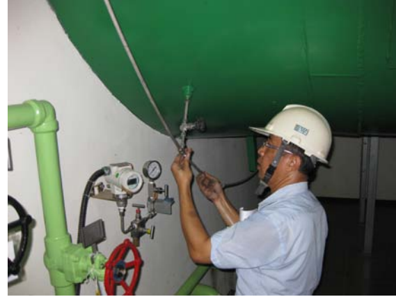
Fig. VI: Manifold for Upstream Pressure
