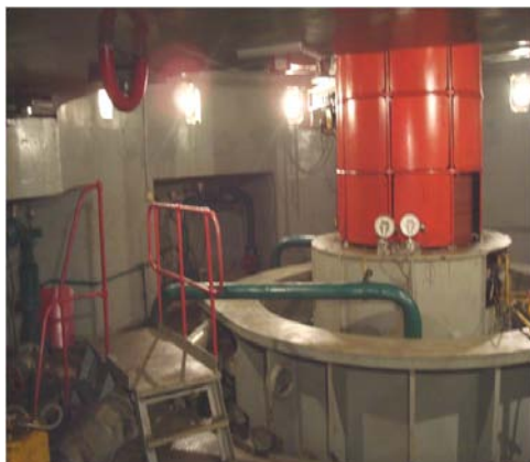
Fig. 5 Dynamic pressure sensors and Static Pressure sensors arrangements
