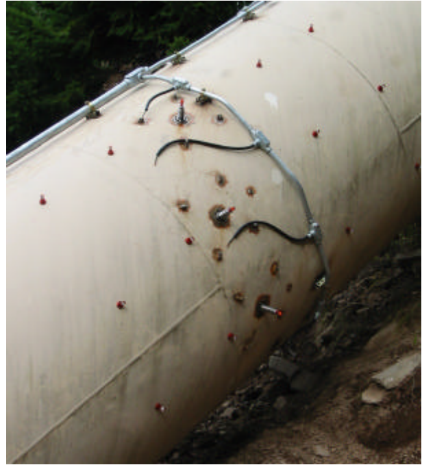
Figure 5: Left; Acoustic transducer with reflecting targets for final measurement. Right; One side of the penstock with 20 reflecting targets and 4 acoustic transducers.
