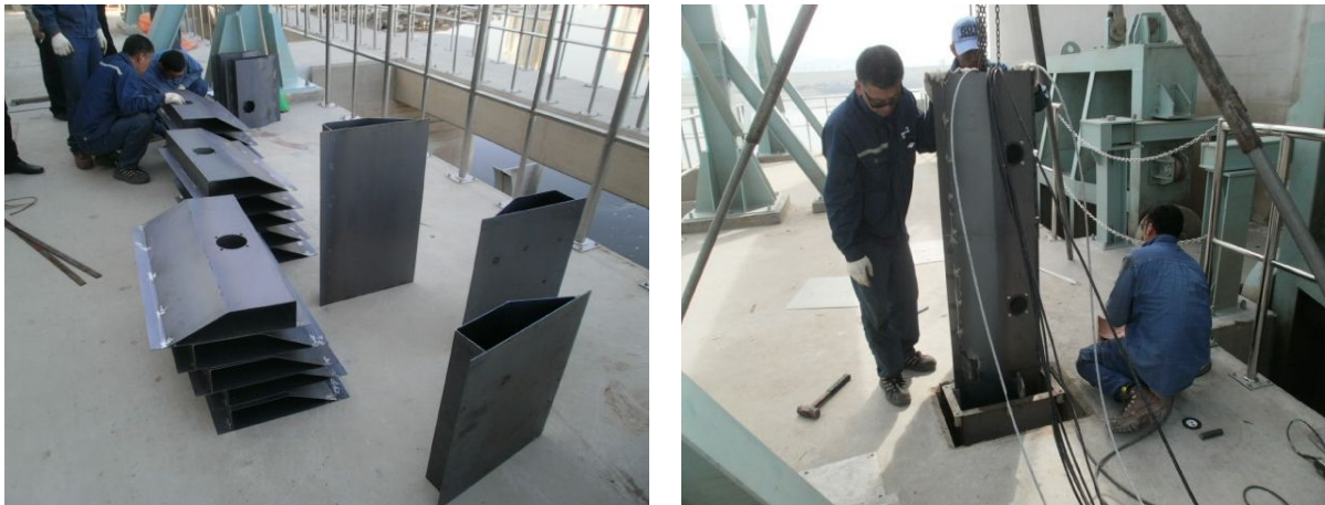
Fig 1 - Frame for the transducers installation
