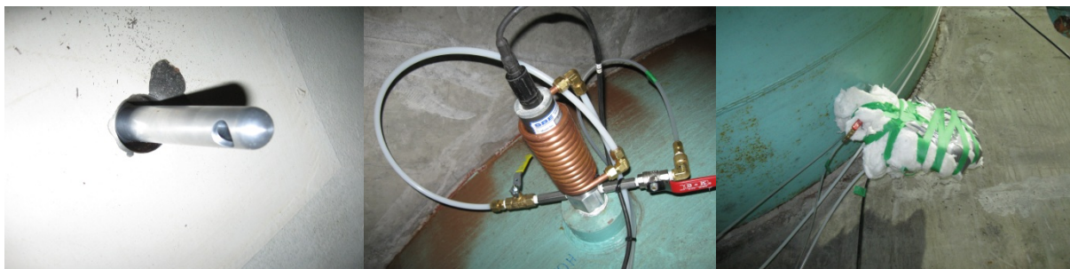
Figure 3: Installation of sampling probe
