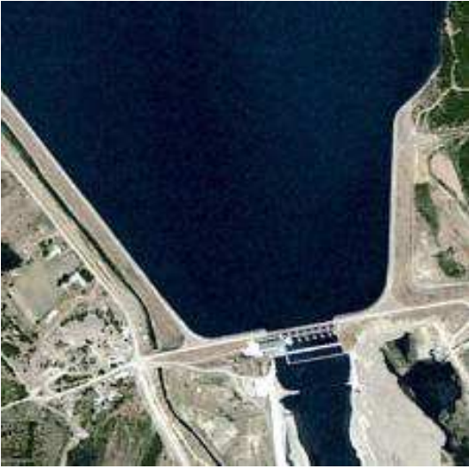
Fig.1 – The HPP reservoir and dam
