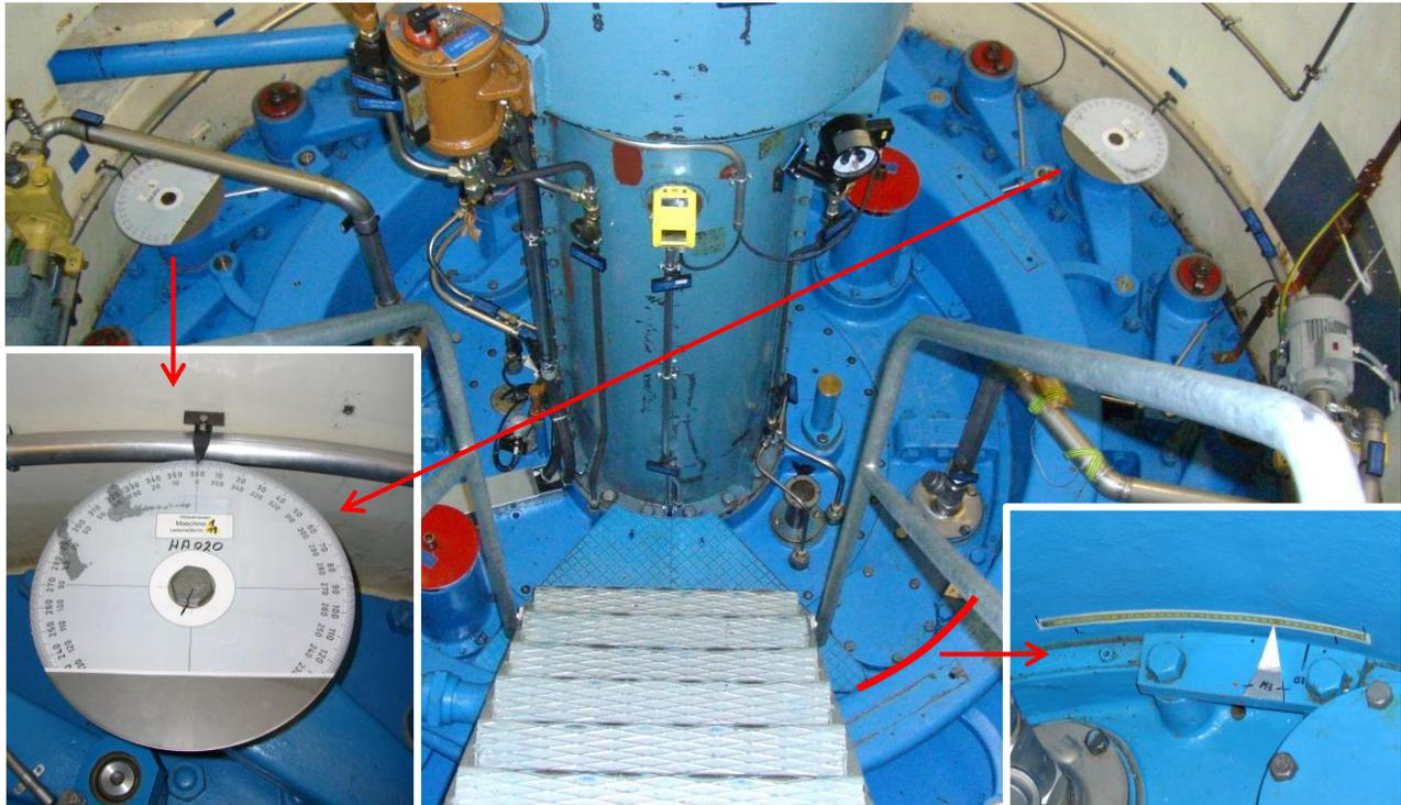
Figure 5 – Position measurements by the regulating ring and the guide vane stem
