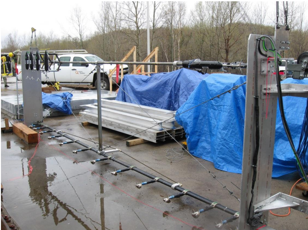
Figure 4: Frame supporting the current meters.
