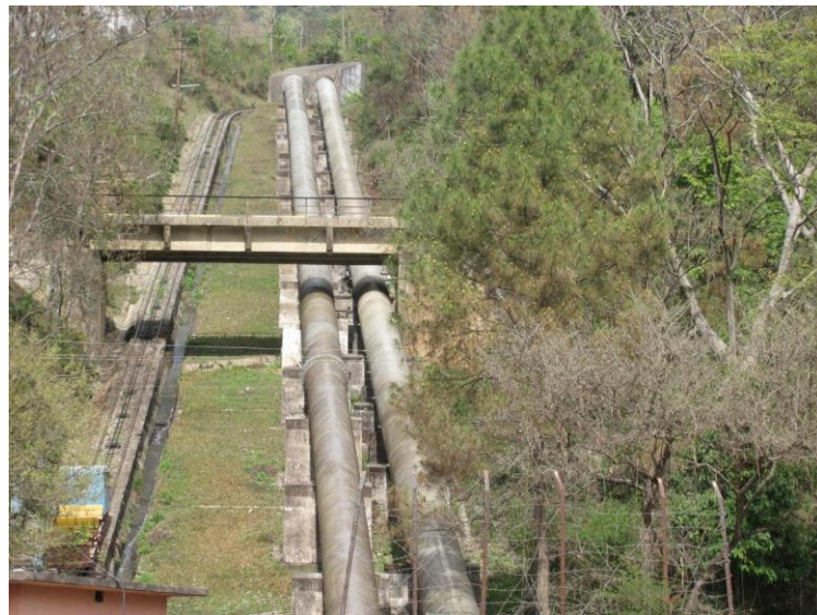
Figure 2 – Two penstocks for Units-1 and 2 and Units-3 and 4
