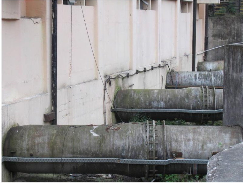
Figure 3 – Individual penstocks for the four Turbines
