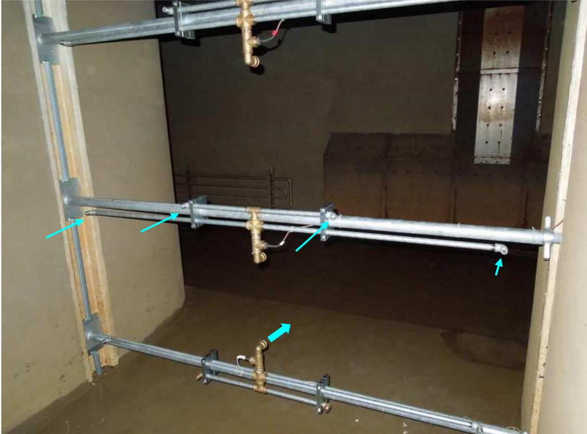
*Fig. 4 Structure with thermometers and collectors in turbine discharge channel*
