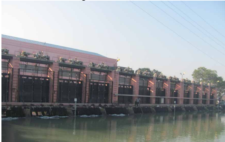
Figure 1 – Twelve intake gates for three units at Mohammadpur Power Plant
