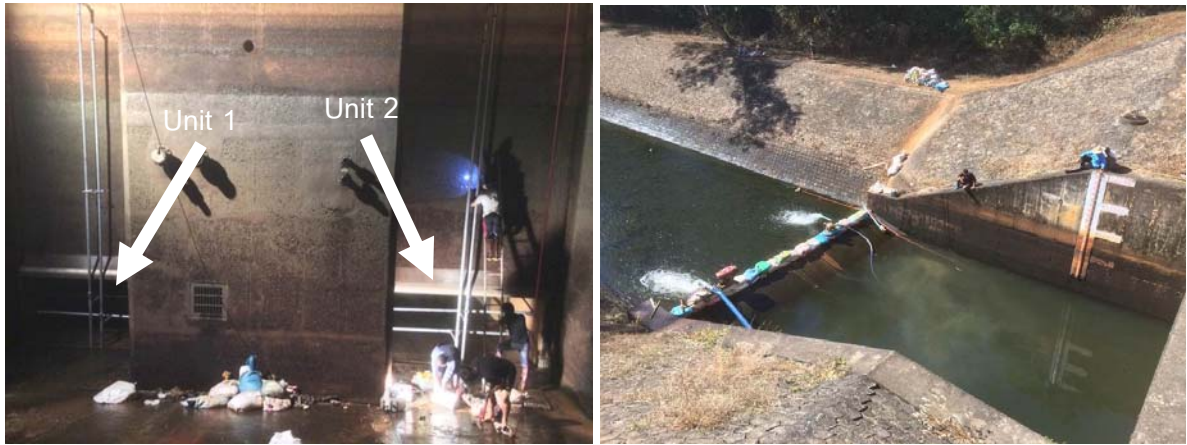
Figure 7: The Installation of Sampling Frame at Draft Tube
