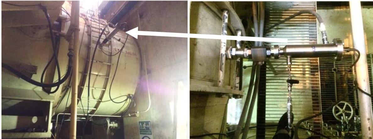
Figure 4: The Installation of Sampling Probe at the Penstock nearby the Inlet Valve
