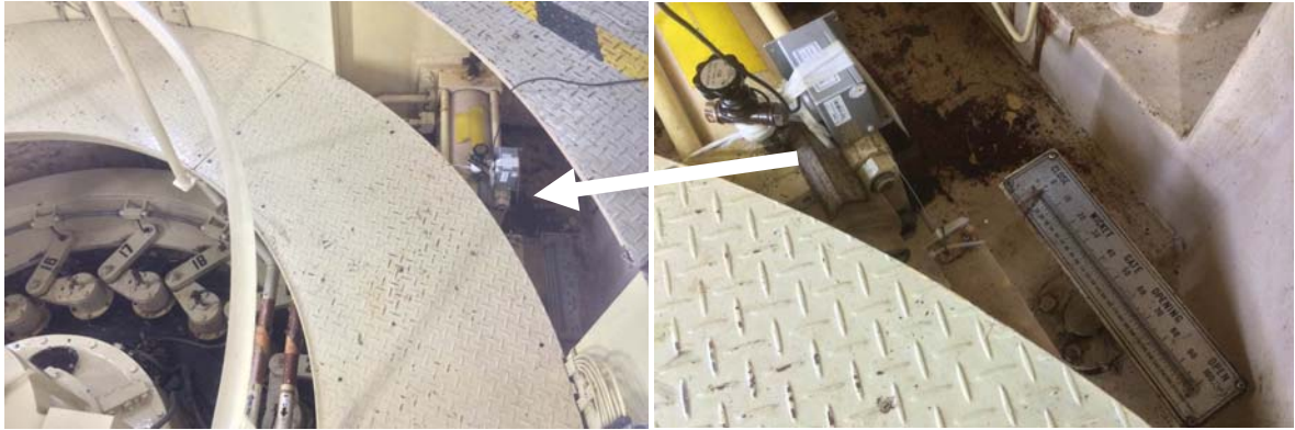
Figure 12: Displacement Transmitter Measuring Servomotor Stroke of Guide Vane Opening
