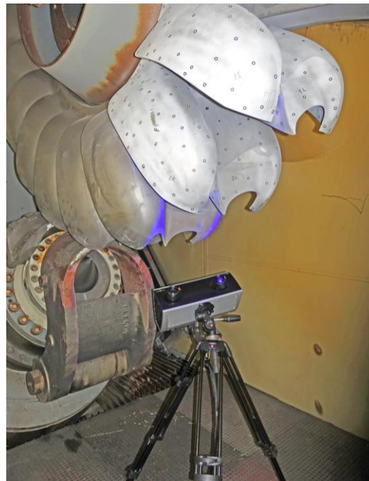
Figure 5: Digitizing of Pelton bucket geometries inside a turbine housing in HPP Fieschertal: camera with projector mounted on a tripod with stick-on reference points on the buckets.
