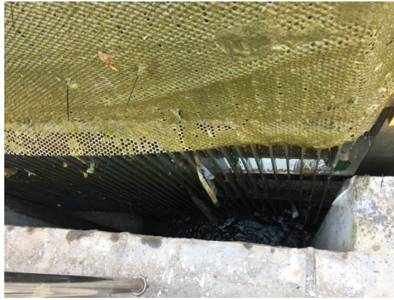
Fig. 12: trash rack with mesh
