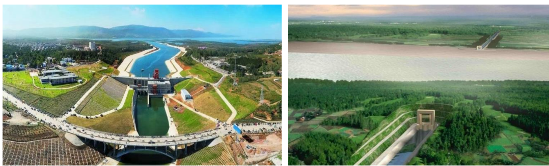
(a) headwork project
