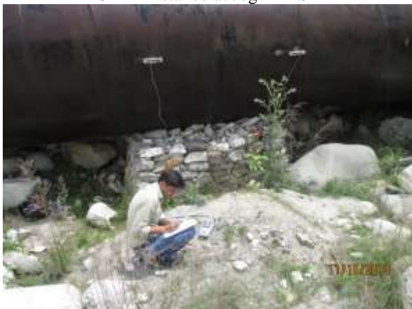
UTTF installed at Gangani Plant
