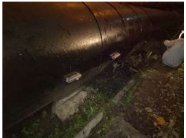
UTTF installed at Periyar IV HEP
