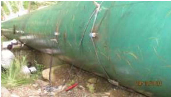
UTTF installed at Lower Nanti SHP
