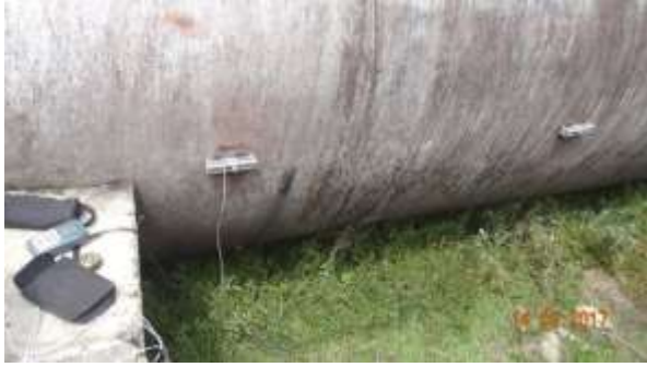
UTTF installed at USHP II SHP
