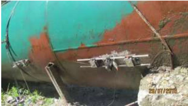
UTTF installed at Jogini II SHP
