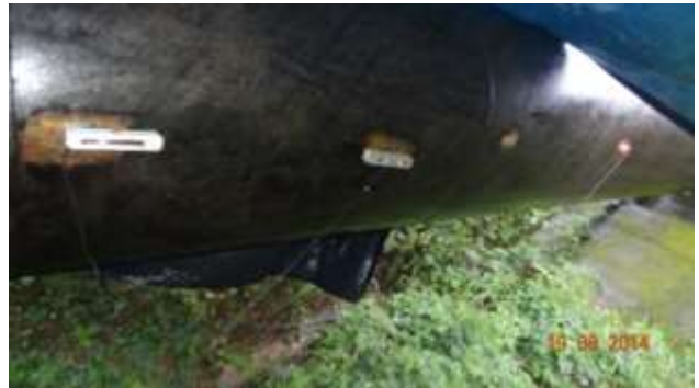
UTTF installed at Phoozhithode SHP
