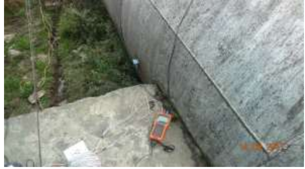
UTTF installed at USHP II SHP
