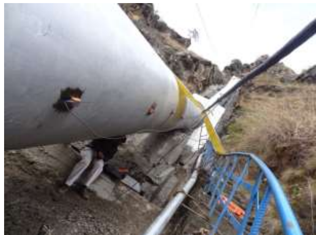
UTTF installed at Ganvi II SHP
