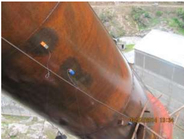
UTTF installed at Ranjha Ala Dunadi SHP
