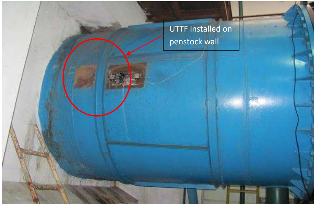
Figure 2: Ultrasonic Transit Time Flowmeter installed on penstock for Discharge Measurement
