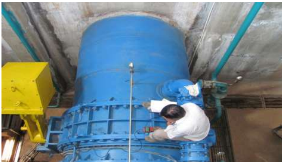
Figure 4: Ultrasonic Transit Time Flowmeter installed on penstock for Discharge Measurement
