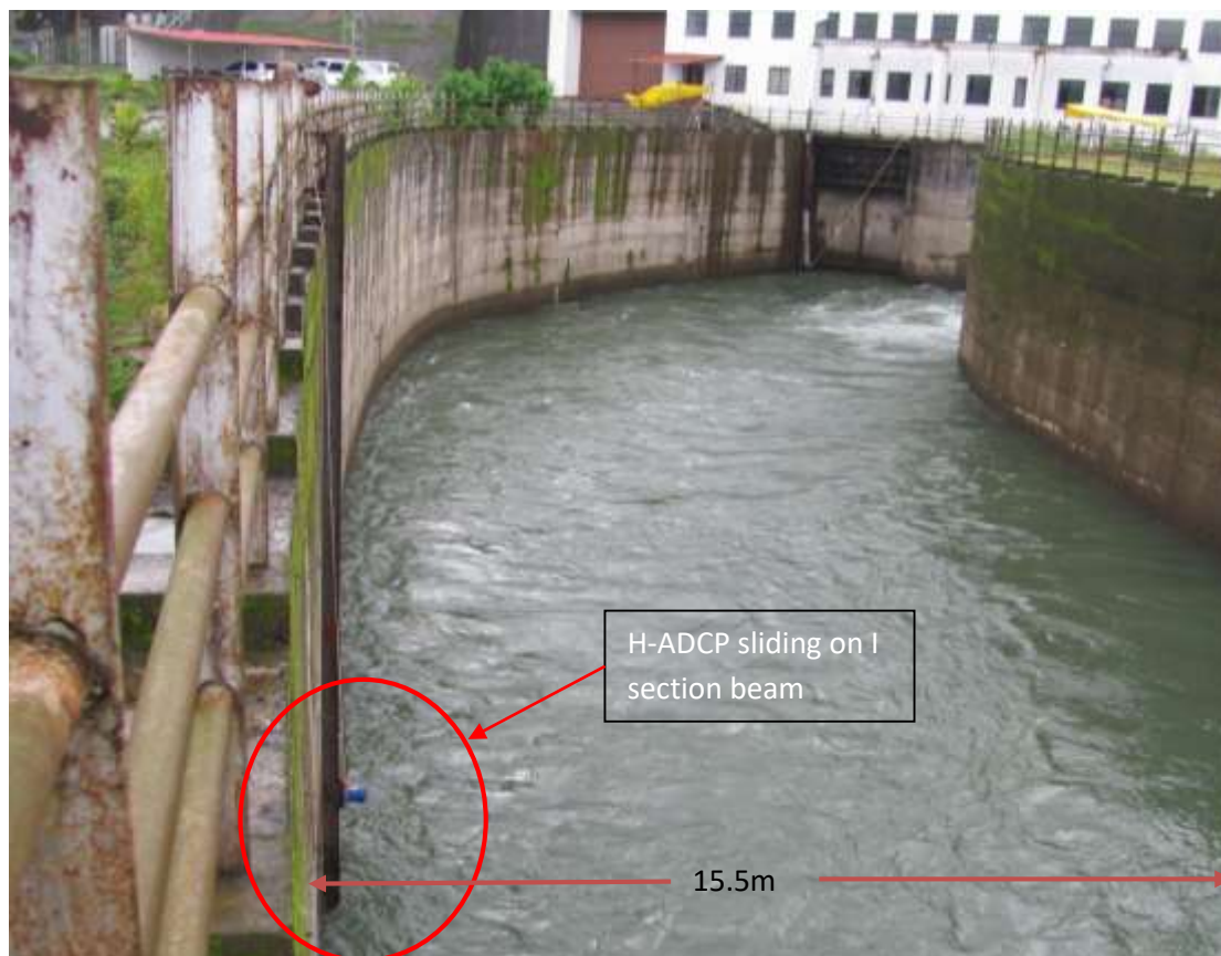
Figure 1: ADCP Transducer sliding on the vertical I-section installed at tairace right side wall for discharge measurement at Radhanagri SHP
