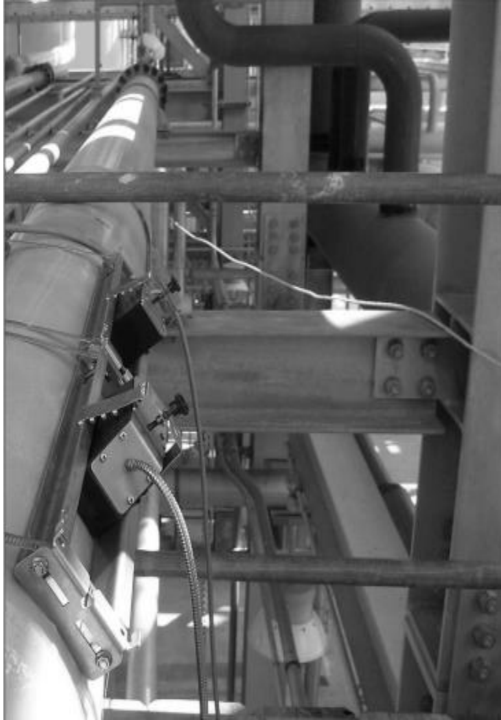
Fig. 1 Ultrasonic Clamp-On Measurement
