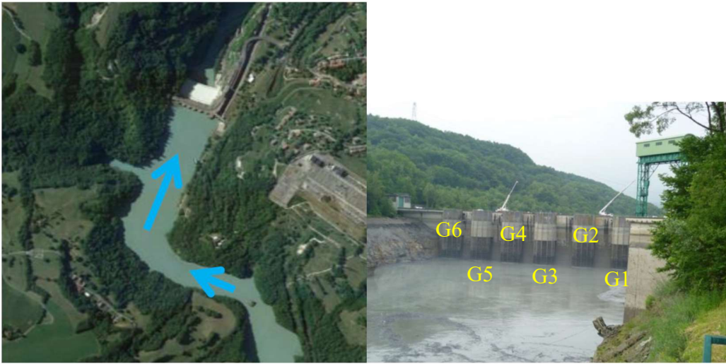
Fig. 5: Genissiat dam seen from upstream.
