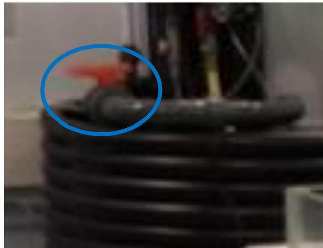
Fig. 3 shows V1 valve, which is a spherical valve used to start the flow in the circuit. It is installed at the output of the upstream reservoir.
