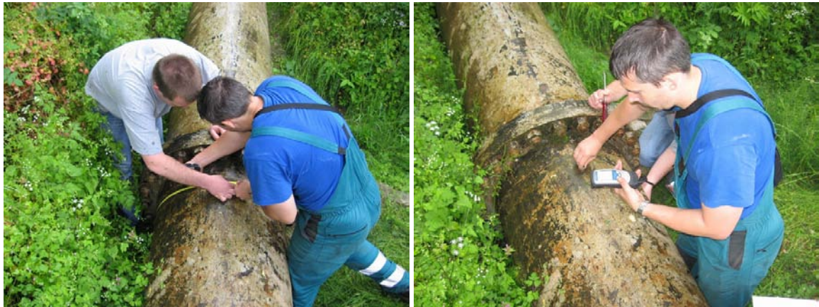
Fig. 5 – Penstock outer circumference and wall thickness measurement
