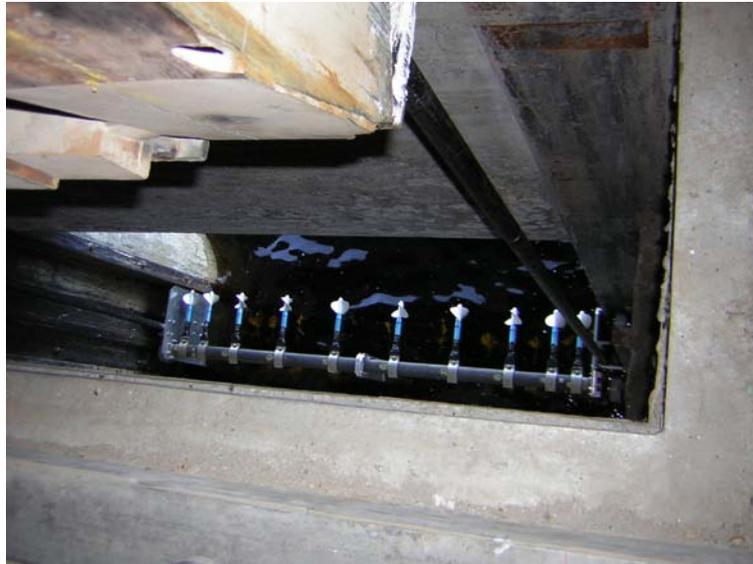
**Figure 19: Moving frame at the intake of the unit**
