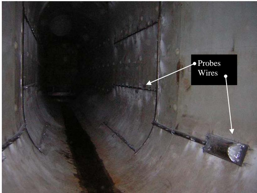
Figure 22: Installation of the transient time acoustic probes.
