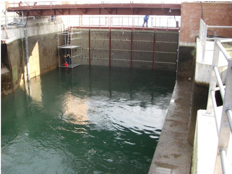
(b) Mounted frames inside the intake channel: The water level in the intake part is equilibrated with the tailrace level. It was not possible to adjust sensor pairs with a laser below the water surface.
