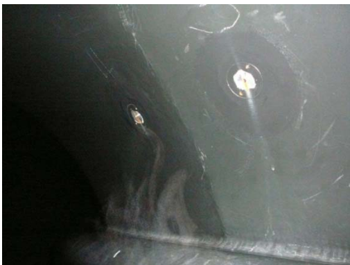
Figure 11: Example of pressure tap installations (good and bad realization)
