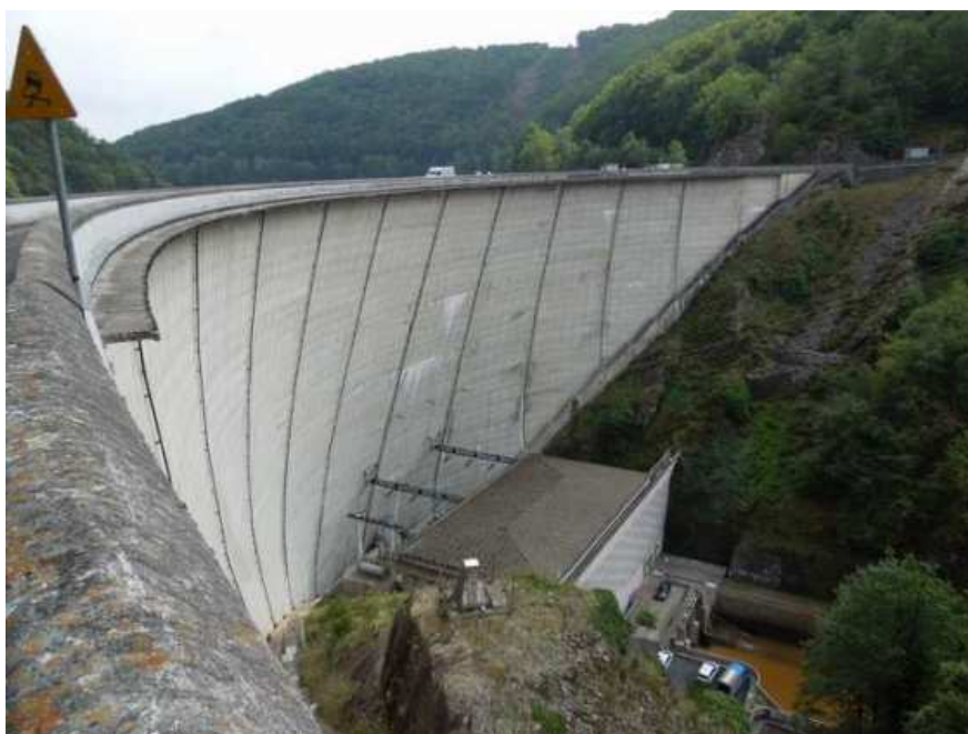
Figure 1 : Dam and powerhouse Enchanet
