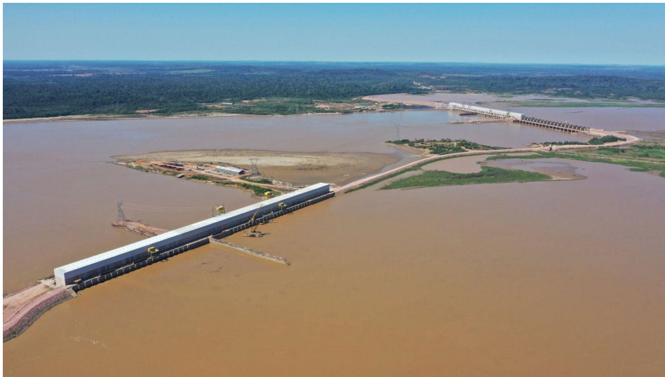
Figure 2: Jirau Hydroelectric Power Plant [6]
