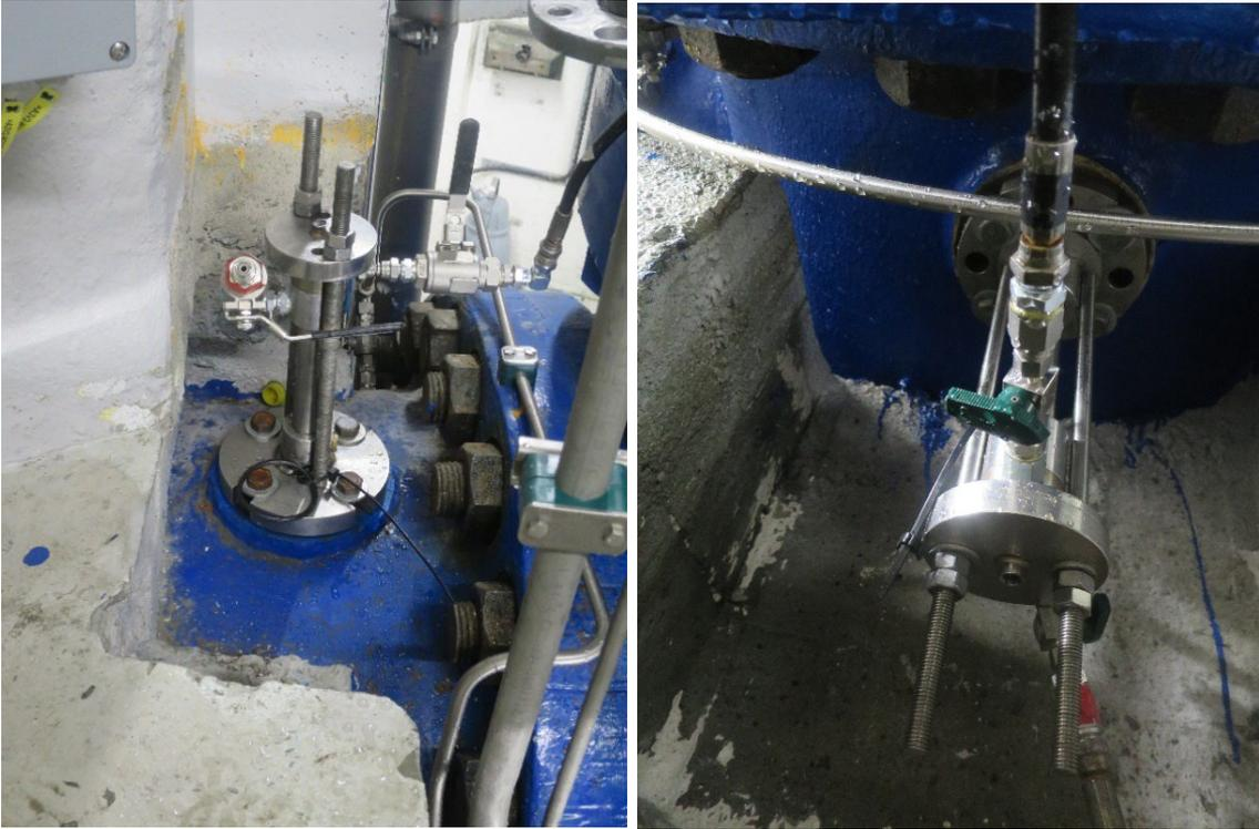
Sampling probe located at top and bottom of spiral casing
