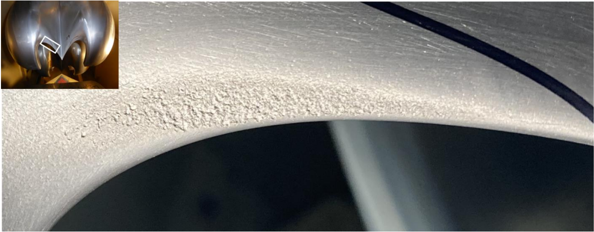
Figure 5: Position and detail image of the cavitation damage on cut-out lip
